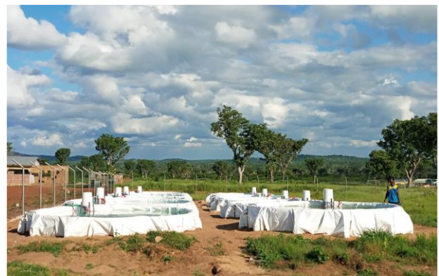
Ten (10) fish ponds constructed for the Bui Power Authority
