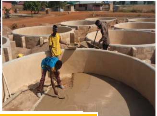
Fish pond construction at Bui in the Brong-Ahafo region of Ghana
