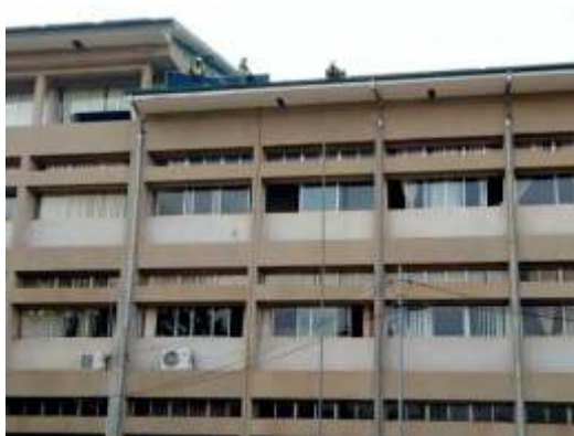
Solar panels being installed at the CRI main building
